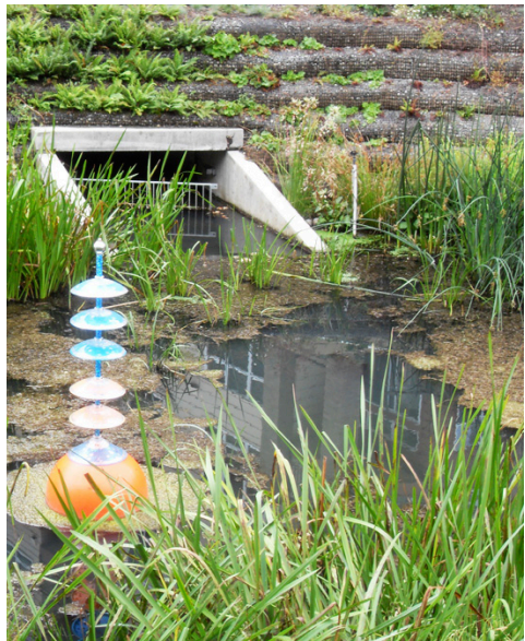
Detail of vegetation in the Thornton Creek Water Quality Channel
