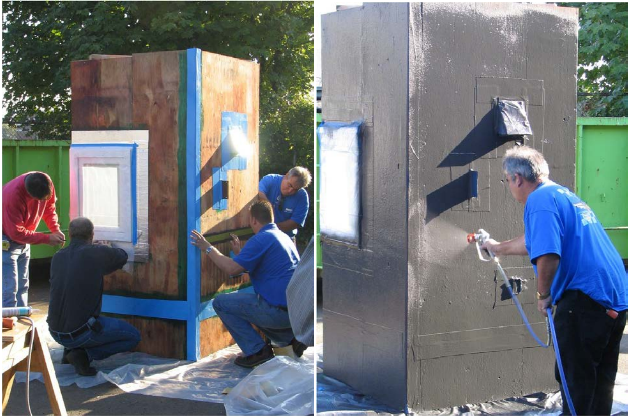
Figure 1. Installation demonstration by basis of design liquid-applied membrane manufacturer.
