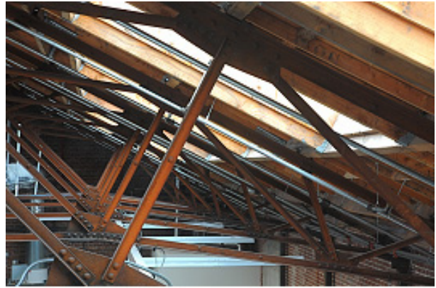
Figure 10: Interior, 3536 Sacramento Street. Photograph by Sharon Risedorph.
