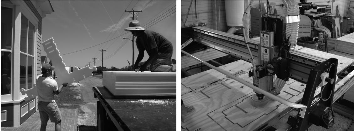
Figure 12 CNC wood router in Exmore Va. And loading a finished building component cut from a sheet of polyethylene onto a truck.
