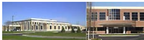
Left: Southshore Surgery Center Exterior Right: Dearborn Medical Building Exterior
