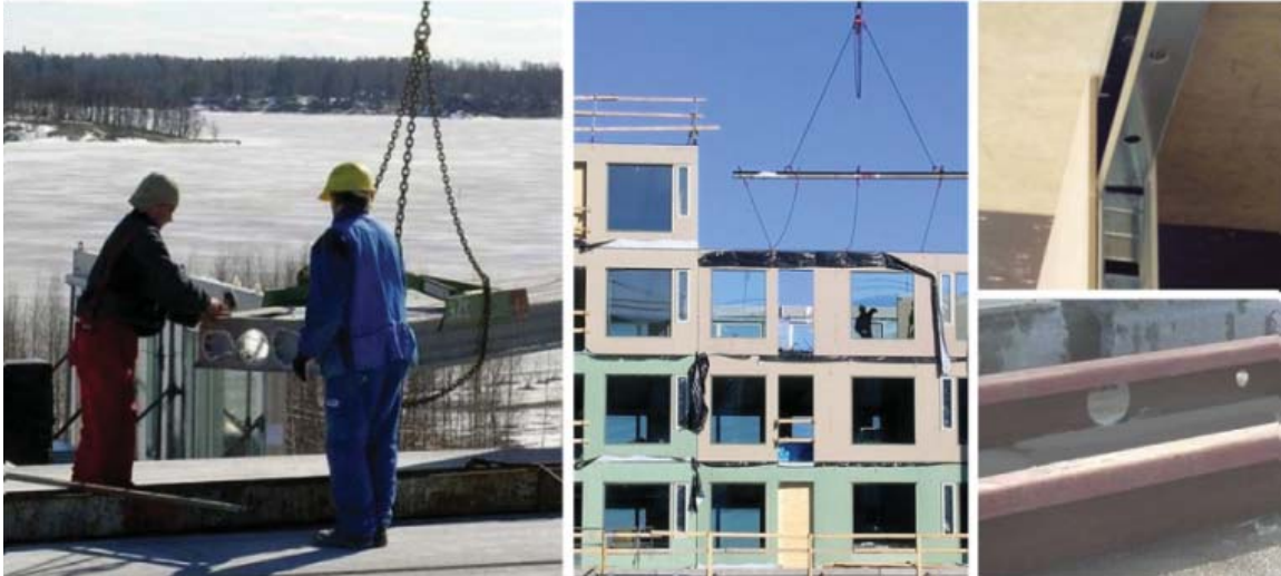
Figure 11: Offsite manufacturing of load-bearing walls minimizes the construction time on site (Image courtesy of Esko Khari and Esko Enkovaara).
