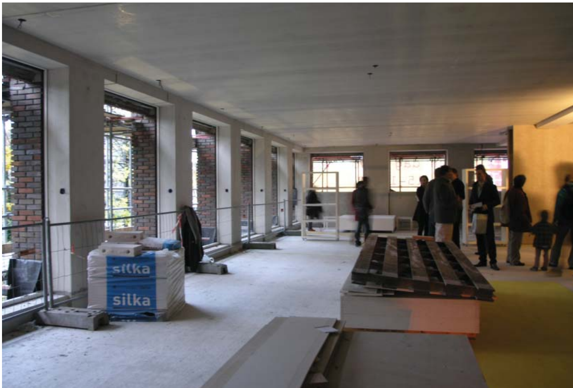
Figure 5: Interior of Solid Oud West under construction.
