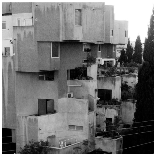
Figure 2: Dubiner Apartment House is a composition of concrete solids, voids and vegetation 16
