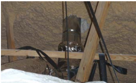
Figure 2: Plumbing penetrations
