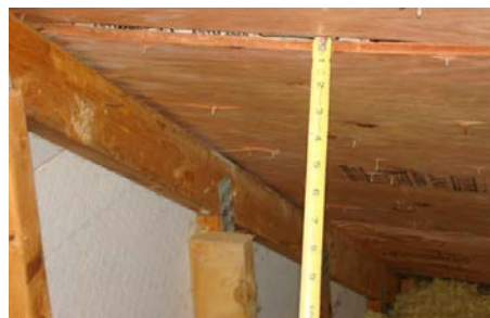
Figure 5: Surface area openings at roof
