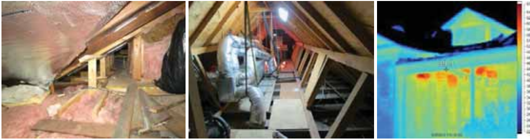
a) poor attic condition in home 3, b) uninsulated attic in home 2, c) infiltration losses in home 2 Figure 1: Sample images from the visual and infra-red inspection of the case study homes.
