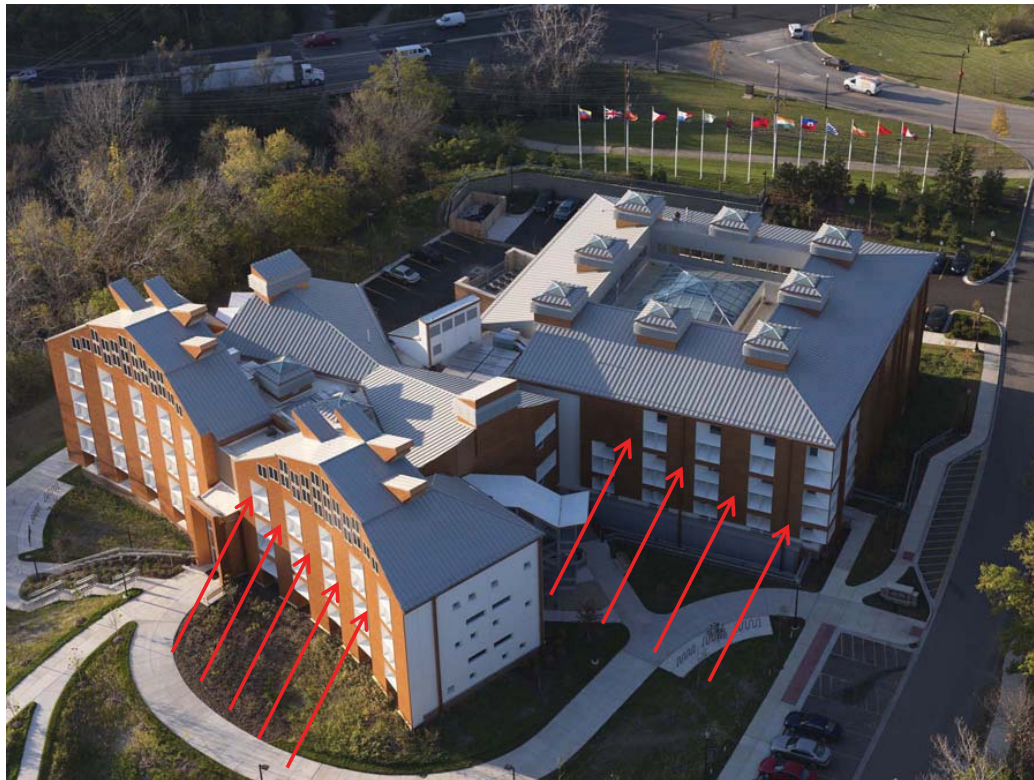
Figure 2: Cladding (arrows) indicates location of stacks for natural ventilation in HAWAC
