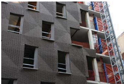
Figure 1: Photograph of 290 Mulberry Street under construction. flickr (Creative Commons): (joevare 2008)
