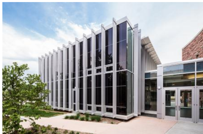
FIGURE 13: Interior and Exterior views of the Morgan Library at Colorado State University where EC glazing has been installed in a modern glass cube design to tame the intense western sun. The interior view shows the glass being controlled in two zones. The upper zone is in the fully tinted state whilst the lower zone is in an intermediate transmission state.
