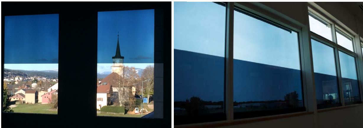
FIGURE 12: Examples of one of the new advances in EC glazing: In-pane zoning. The left image shows an EC product installed in a building with the top of each pane in a tinted state and the bottom of the pane in a higher transmittance state. The right image shows panes split into two zones, the lower part fully tinted and the top part partially tinted. Photographs courtesy of SAGE Electrochromics, Inc.
