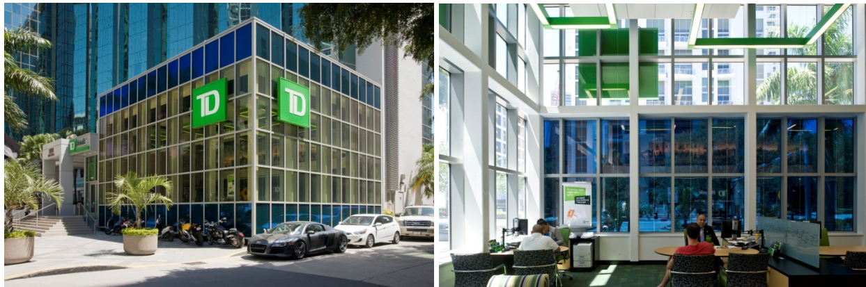
FIGURE 14: EC Glass installed in a glass cube design for a bank on Brickell Avenue, Miami, Florida.
