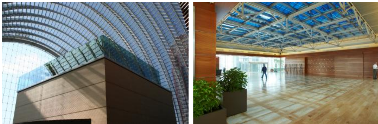
FIGURE 17: The exterior and interior views of the Dorrance H. Hamilton roof top garden in the Kimmel Center for the Performing Arts. EC glass is used in the roof to control the heat gain and provide a comfortable space year-round.
