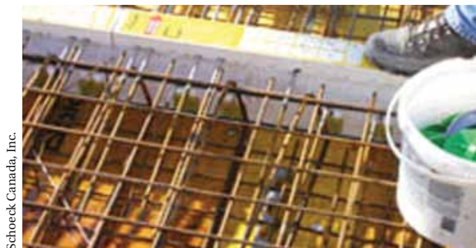
Figure 5. Pre-manufactured thermal break. High-density graphite-enhanced expanded polystyrene. Note the reinforcing rods penetrating the foam are stainless steel, not carbon steel. Stainless steel has less than half the thermal conductivity of carbon steel.
