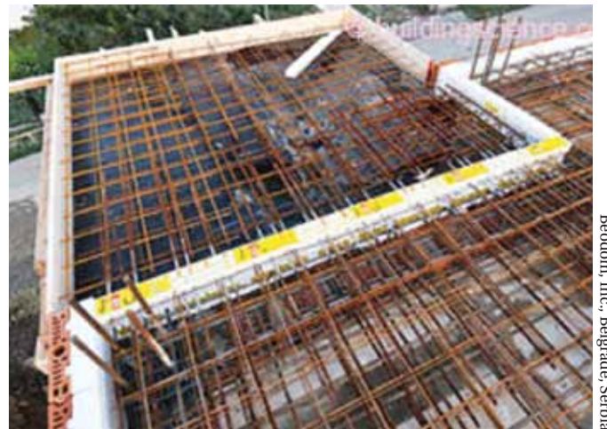
Figure 6. The product shown here, which is being used on a building in Serbia, prevents thermal bridges on balconies.
