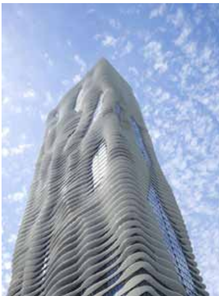
Figure 1. Extended finned-surface, made of concrete.
